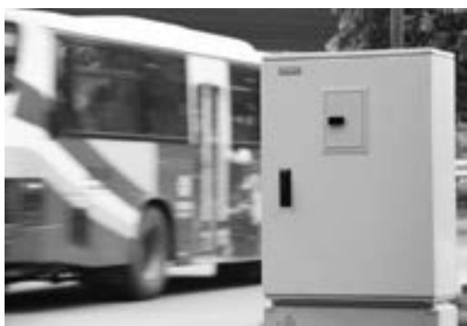
▲ Traffic signal control cabinet is installed by Siemens Corporation
